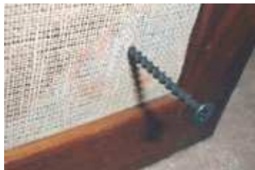
Fig. 2.3. Using a drywall screw to remove the grille.
